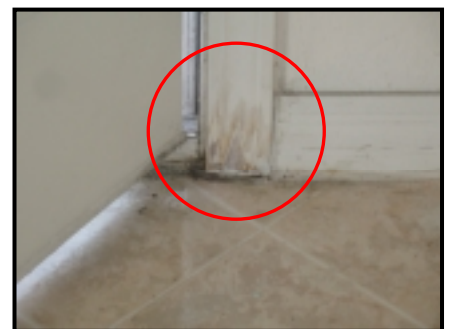
Front door wood trim.
